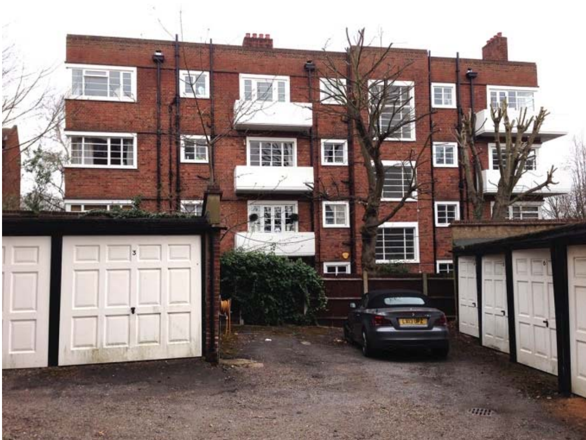
Photo C – View of Emmerson Court
